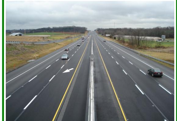
Pennsylvania Turnpike Cumberland County 6-Lane Widening
