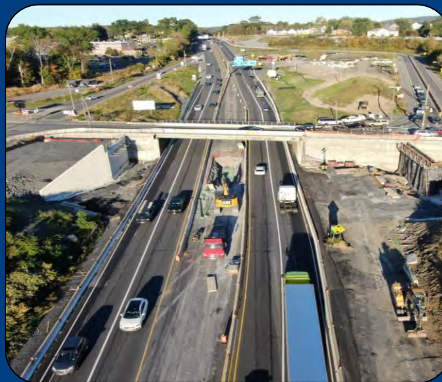
SR 80 Realignment and Bridge Replacement
