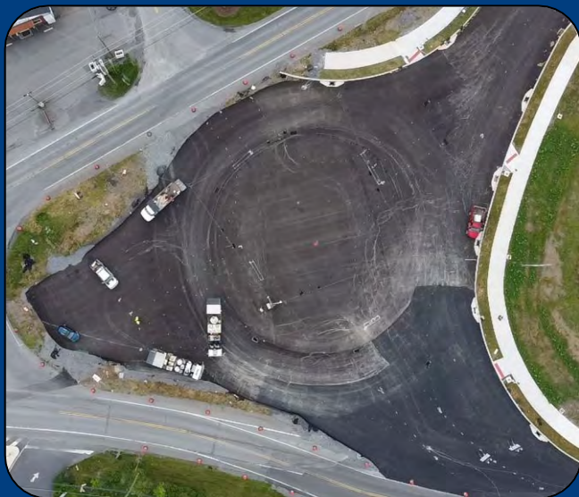
SR 209 Realignment and Roundabout Construction
