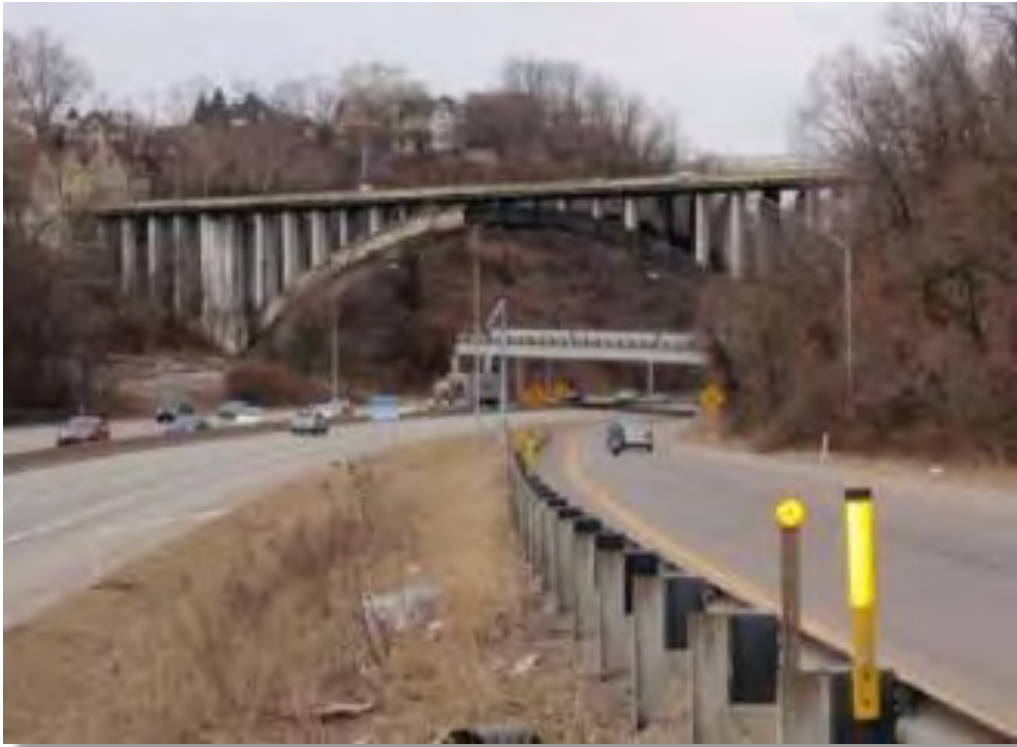
Greenfield Ave. Bridge City of Pittsburgh
