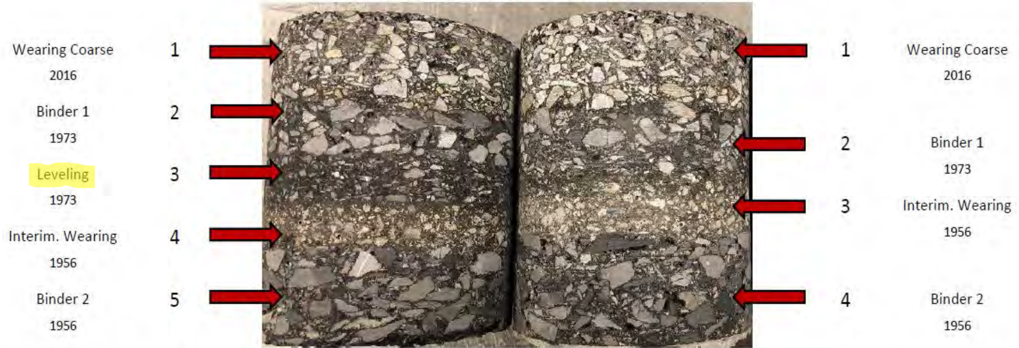
Right Wheel Path Core Example of Differing Bituminous Layers Center Lane Core
