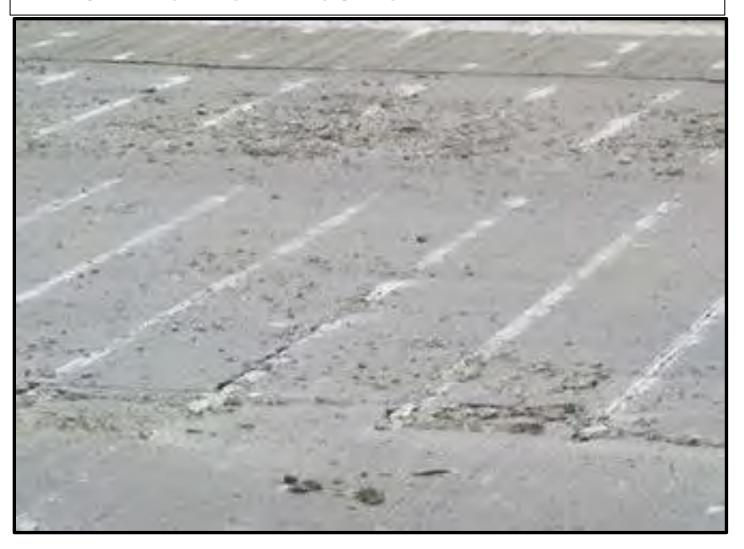
TYPICAL CRACK & SEAT PATTERN – MAKES A GOOD BASE
