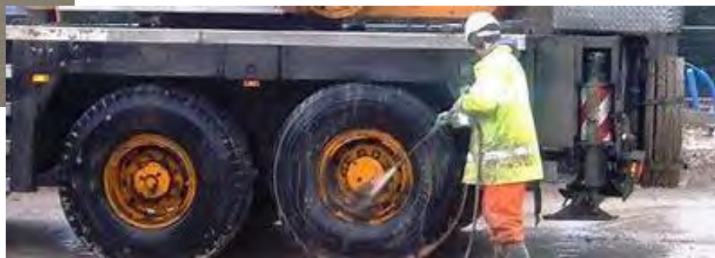
Wheel Washing to Remove Sediment
